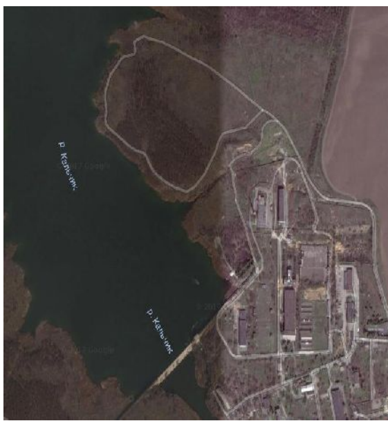
Fig. 2. Starokrymsk filter stations 1, 2 Enterprise «Voda Donbassa»
