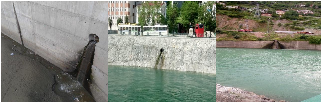
Figure 2. Artvin city center wastewater discharge points
