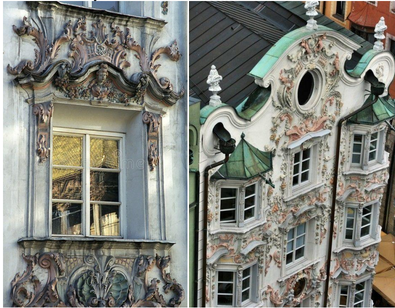
Picture 1. Framing for windows
