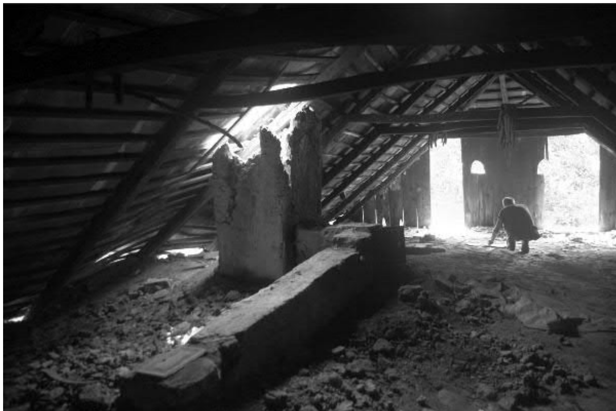
Fig. 5: Koromľa (Slovakia, Sobrance District), Nr. 114, the loft with the smoke shaft and chimney (photo by M. Volovár 2018).
