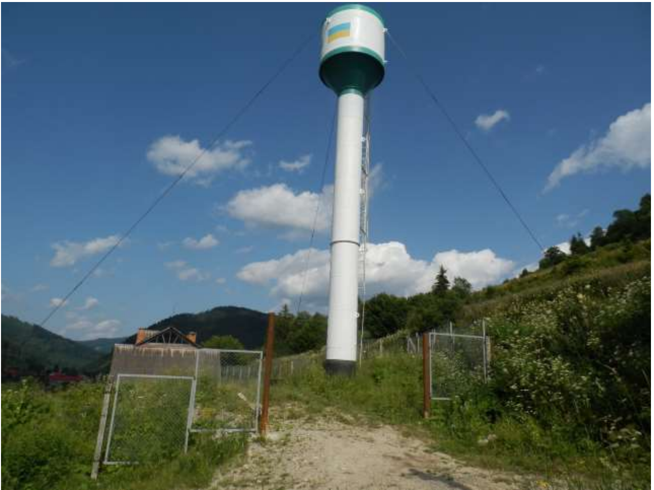
Fig. 1 General view of the surveyed structure.
