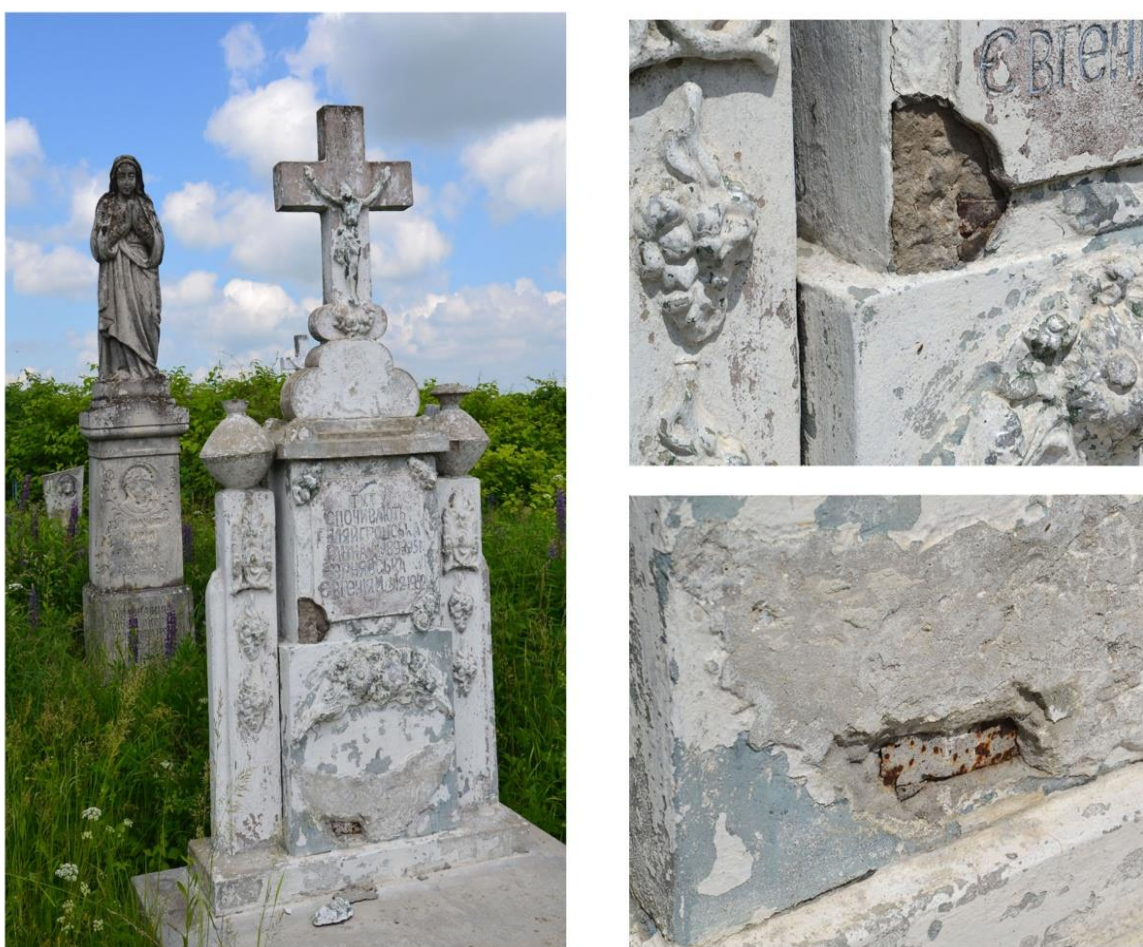
Fig. 2. Destruction of a monument made of reinforced concrete
