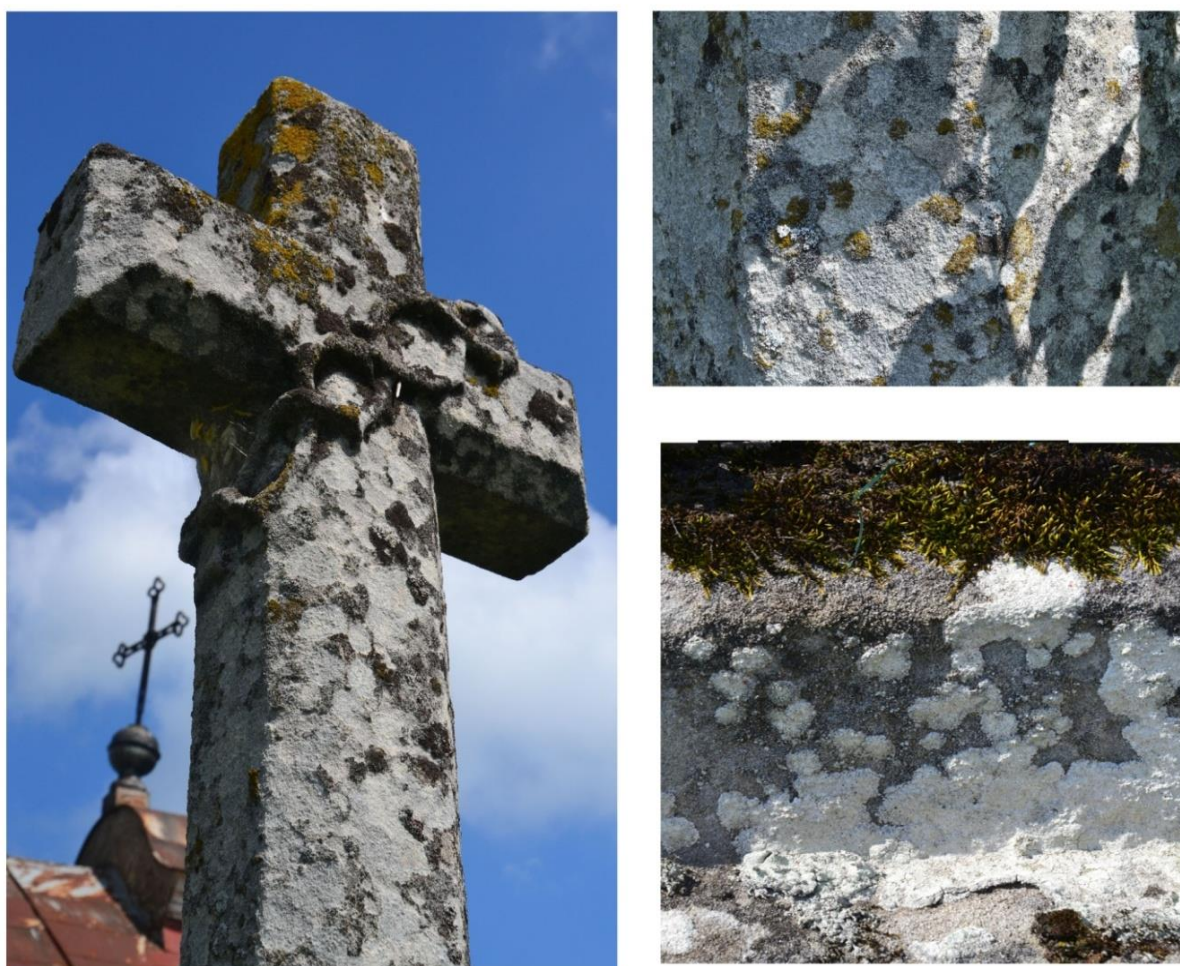
Fig. 1. Biogrowths and the destruction of stone caused by them on the cross from the cemetery in Pidkamen
