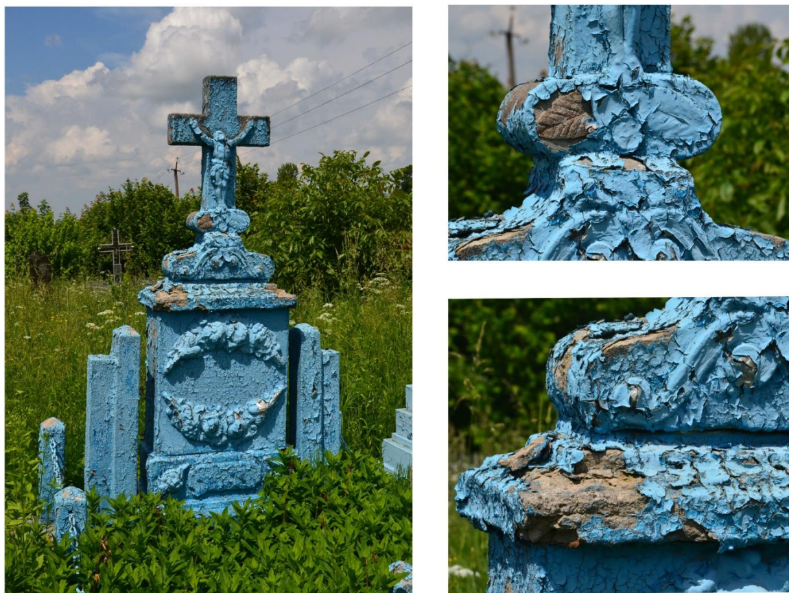
Fig. 3. Destruction of a stone covered with oil paint
