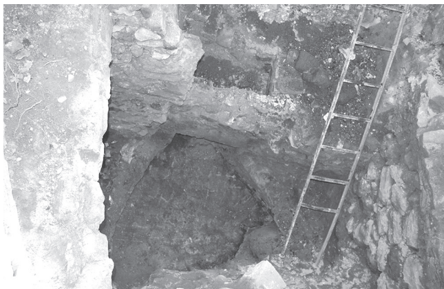
Fig. 5 Collapsed arch
