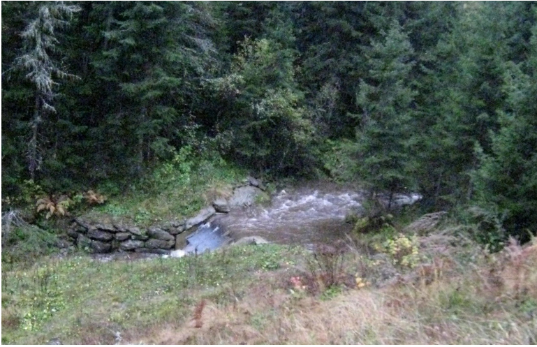
Photo 1-1. Dam on a stream without pondage for micro HPP in the Alps (October 10, 2013, South Tirol, Italy).
