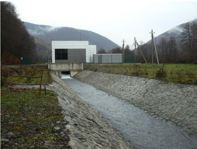
Photo 9-5. The canal from hydropower plant: site No 7.
