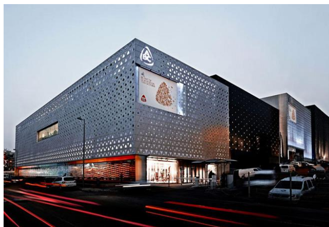
Pic. 1 ABC Shopping Center, Lebanon. The basis of the facade design is perforated metal panels with various perforation patterns
