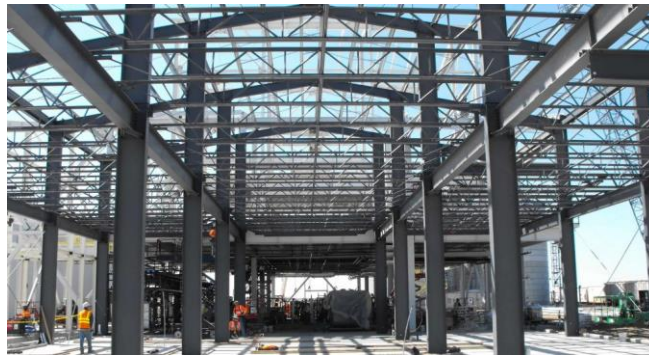
Pic. 3 Spatial framework of a retail facility
