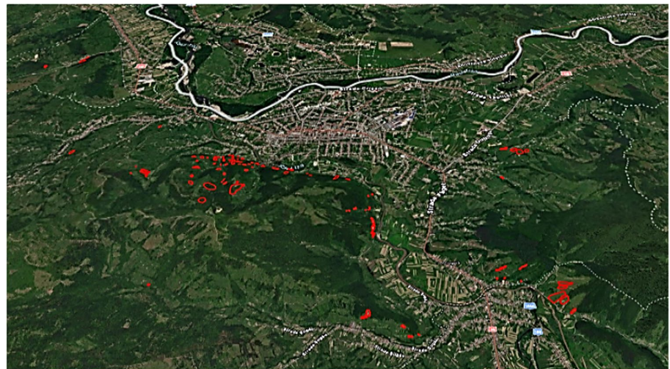
Fig. 7 Land layout of landslides in the area of Sighetu Marmăției Municipality, 120 identified cases (Source: GeoSES Project (Project GeoSES 2021))
