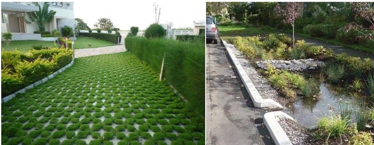
*Fig. 9.4. Parking lots with water-permeable surface and a rain ditch (Photo from the Internet)*
