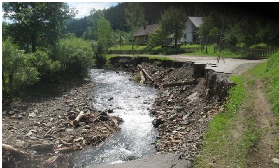
Fig. 10.1.2. Road in Lopushne village, destroyed by the lateral erosion
