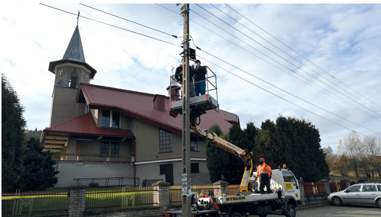
Ill. 2.2. Modernisation of the architectural illumination of the church facade in Sopotnia Wielka in 2020, with the use of a contour light cut-off system. Source: https://ciemnieniebo.pl/pl/dzialania-w-polsce/343-wymiana-oswietlenia-wokol-kosciola-w-sopotni-wielkiej
