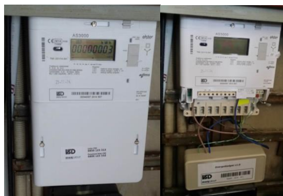
Figure 11. Mounting of the communication module
