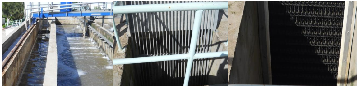
Figure 2: Mechanical pre-treatment steps: a) oil separator sand trap. b) Rake coarse. c) Rake coarse fines
